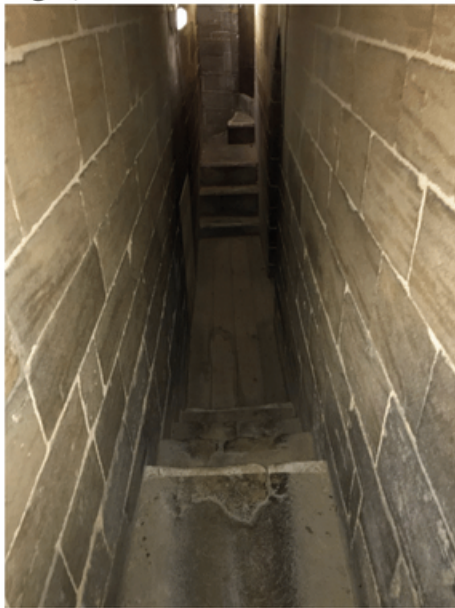
Narrow passage and steps inside bell tower.
